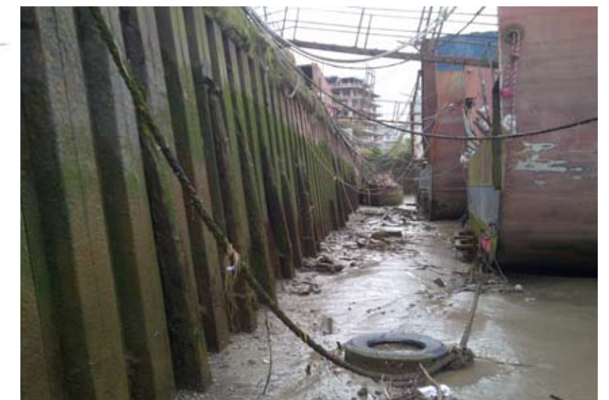
Existing view of sheet pile wall to south. This will be cutdown to form reed bed margin with new flood defence wall to rear
