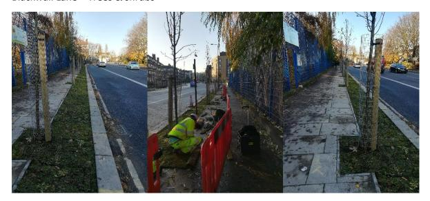
There is now a drainage ditch with little squares coming off it next to the raise, and there has been some work on the school site to install a drainage tank. Trees will be planted in the squares to drink some of the water with overflow going into the drainage tanks under the school car park. Eight new street trees will be planted and in between the street trees will be street specific wildflower meadow. Owen Davies at the council has been very helpful with this initiative.
